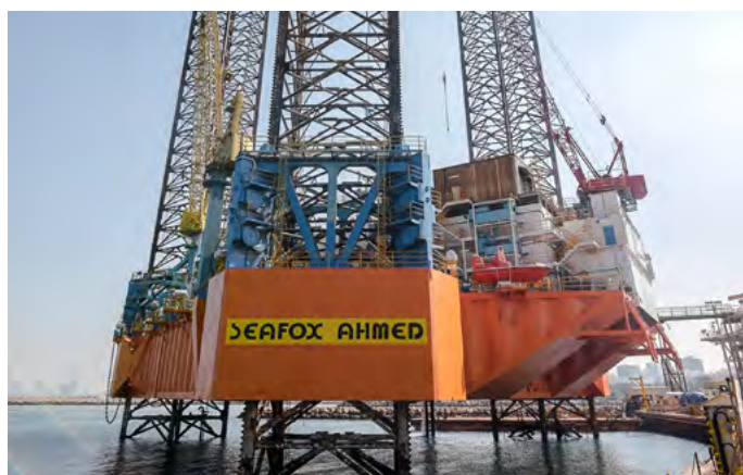
Phase 2 of upgrade work on Seafox "Ahmed" have been completed
