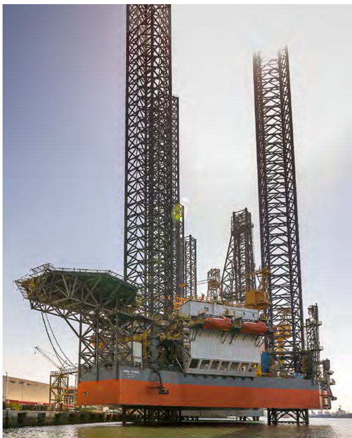
Jindal "Pioneer" back for refurbishment work
