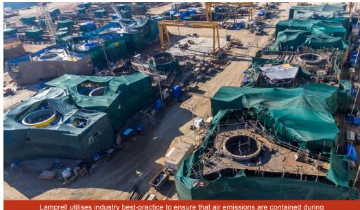
Lamprell utilises industry best-practice to ensure that air emissions are contained during blasting and painting works
