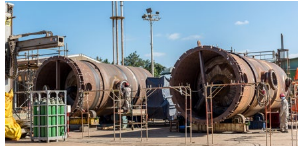
Lamprell is fabricating multiple pressure vessels in its Sharjah facility
