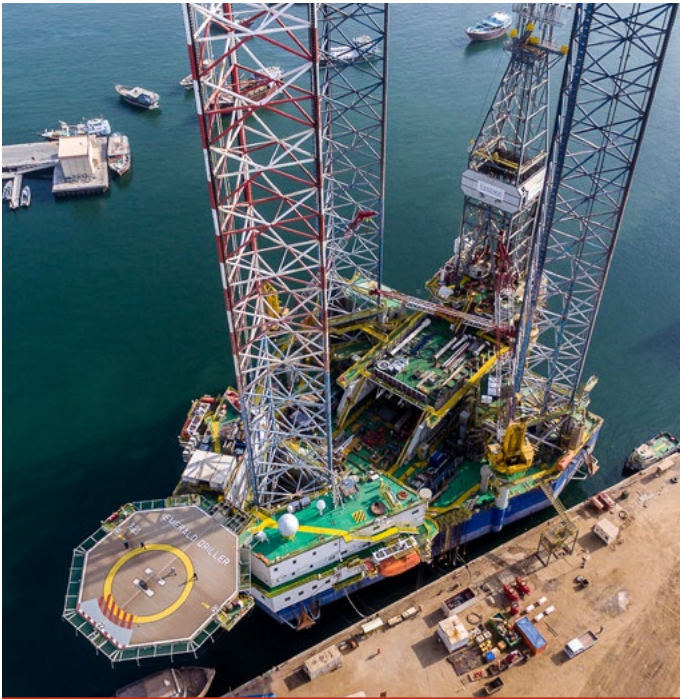
Lamprell successfully completed refurbishment work to the rig “Emerald Driller” which sailed away from our facility in November 2016
