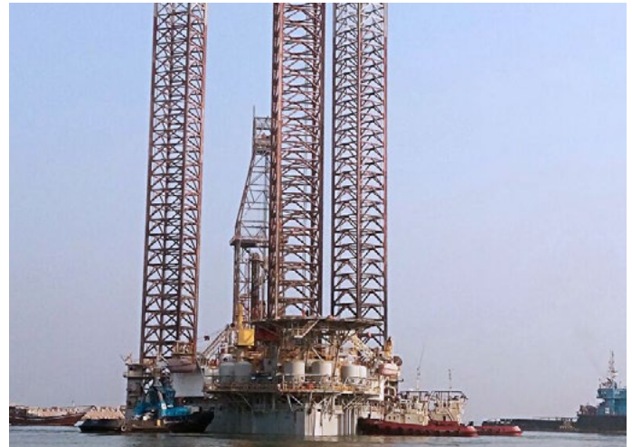
Paragon’s rig “M1162” was successfully refurbished in November 2016
