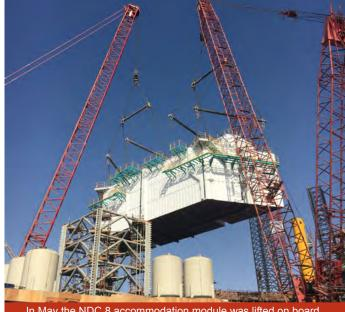
In May the NDC 8 accommodation module was lifted on board the rig and installed successfully
