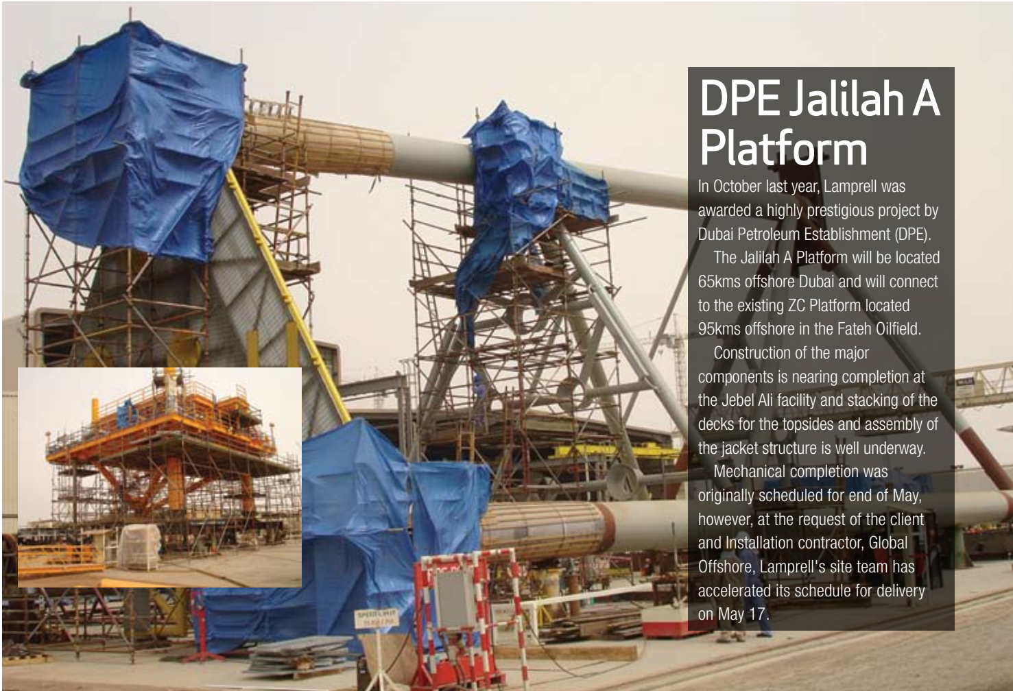
Jacket and Topside deck nearing completion
