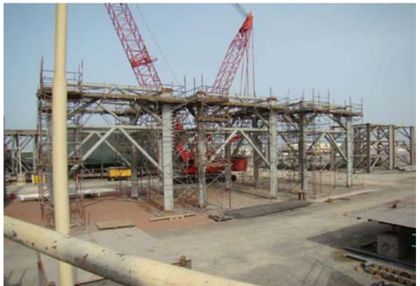
Muhaiymat's leg sections under fabrication
