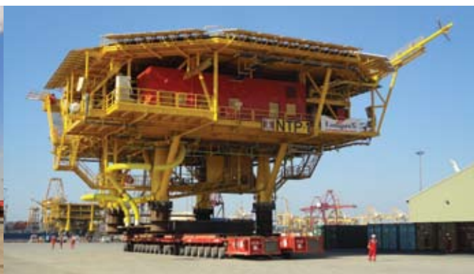
Loadout of ONGC NTP1 and NTP-2 Decks
