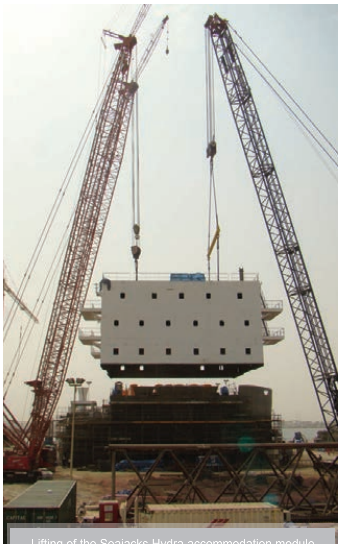
Lifting of the Seajacks Hydra accommodation module
