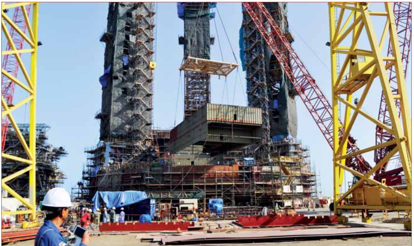
Lifting the 106 MT galley office block into its final position
