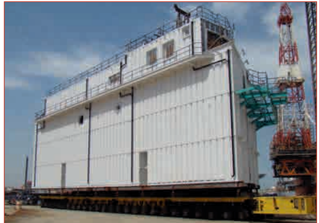
Accommodation block being moved into the NDC rig on 6 May
