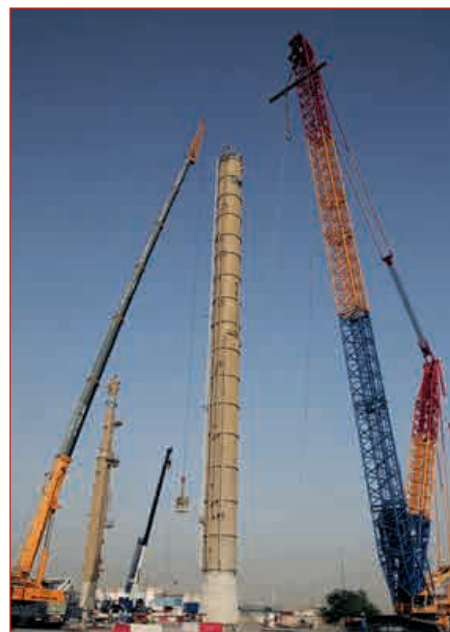
A 501 E – Deisohexanizer column was successfully lifted at the Gulf Refining Company (GRC) process plant in JAFZA by the Engineering & Construction group
