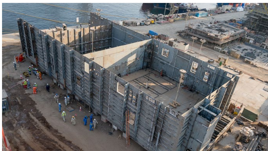
The NDC 9 keel was successfully moved to the vacated Ensco 140 slot in our yard in order to complete the remainder of the assembly phase
