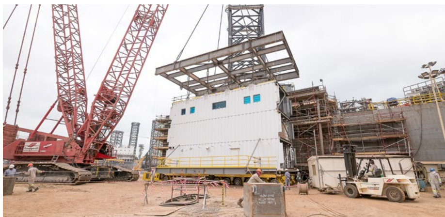
Pictured is Shelf 1 which recently had the accommodation module lifted into position
