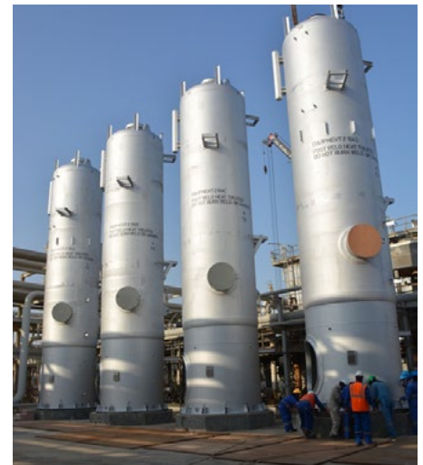
Installation of molecular sieve vessels was completed successfully
