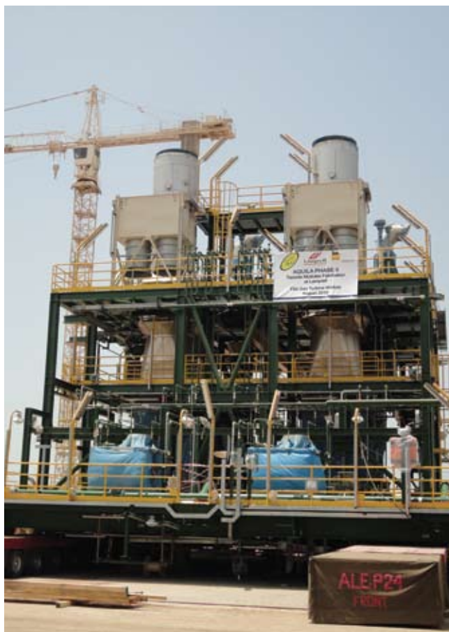
Multi axel trailers in place under the modules in preparation for load out
