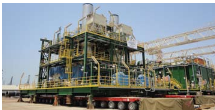
Multi axel trailers in place under the modules in preparation for load out
